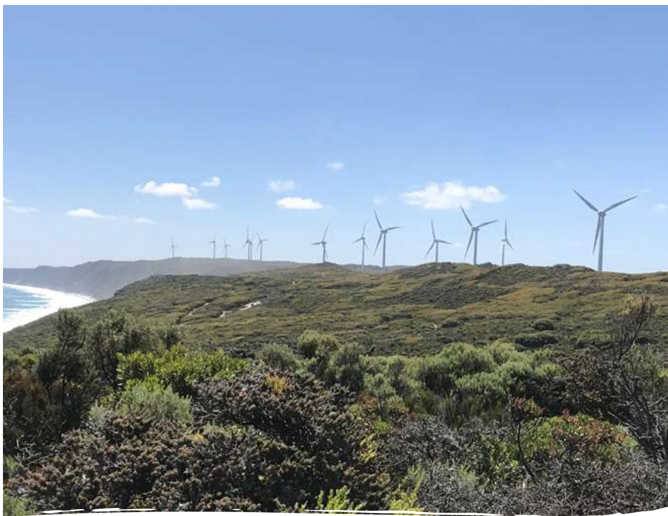
Albany Grasmere Wind Farm, for which Worley has been providing operations and maintenance services since 2018.
